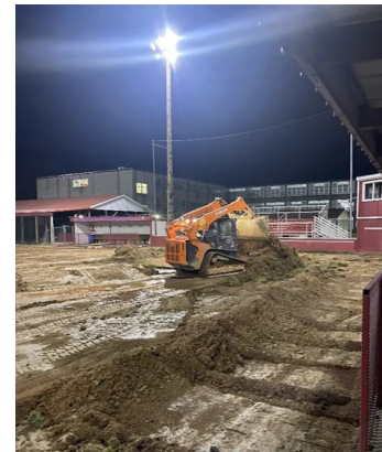
Construction begins on new turf field
